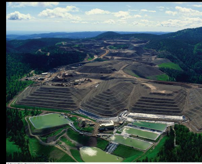
Gold Mine with Cyanide Leach Piles and Ponds in South Dakota, U.S.
